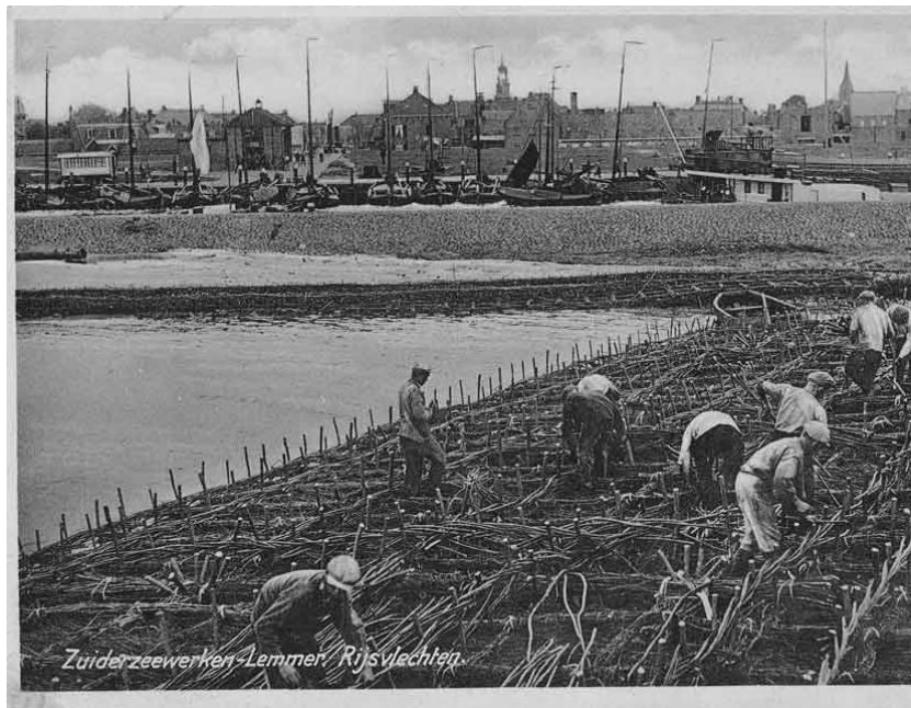
Weaving of willow branches as the base for the sea dike near Lemmer- ca 1935
